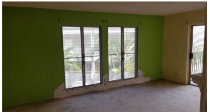
Apparent Defects, Damages, Deficiencies - Walls and Ceiling - Peeling Paint
