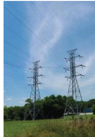
Site Influence - View - Power Lines
