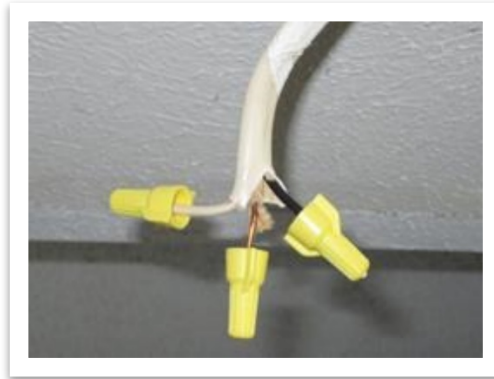
Example of Capping Wires
