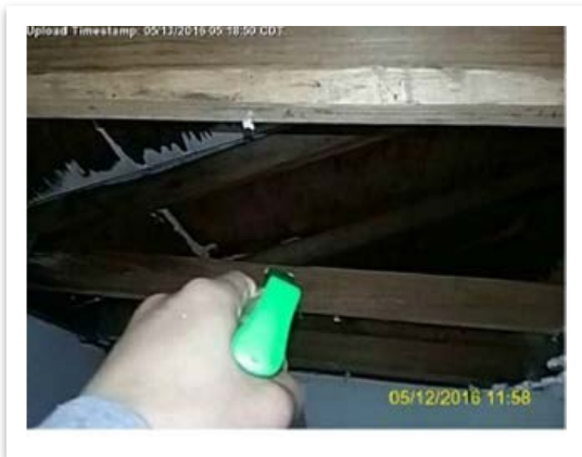
Treatment of studs with antimicrobial solution.
