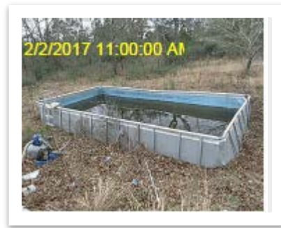
Pool must be drained and dismantled.
