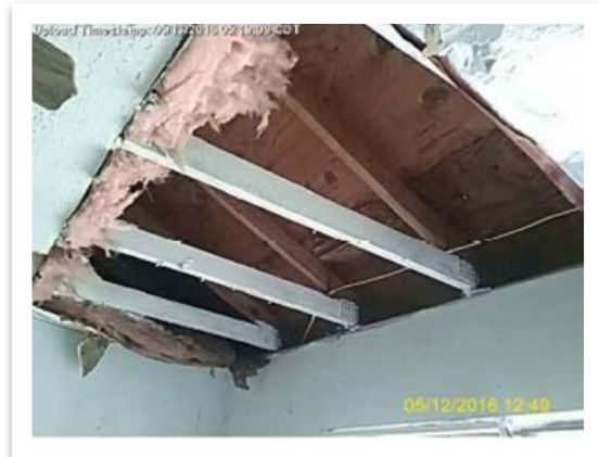
Treatment of studs with stain blocking primer.
