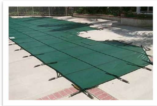
In-ground Pool: Covered correctly.
