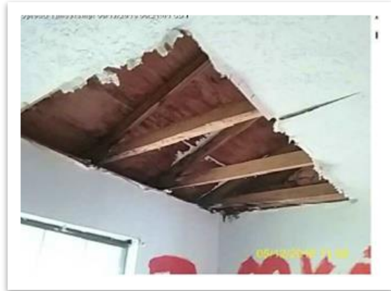
Removal of drywall and insulation.
