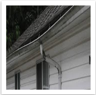
Section of gutter needs repair.
