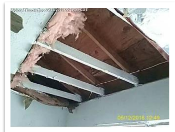
Treatment of studs with stain blocking primer.
