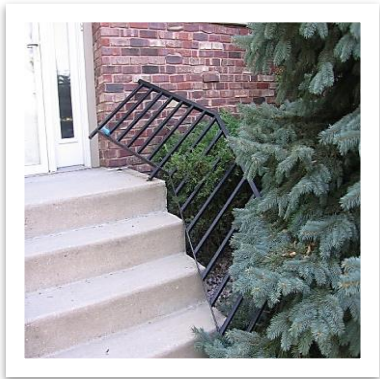
Re-secure handrail.
