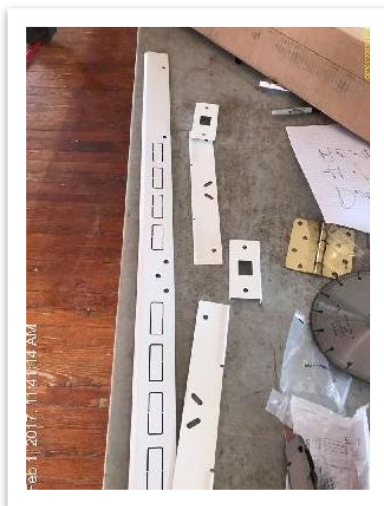
Photo showing door jamb and hinge protection product materials ready for installation.
