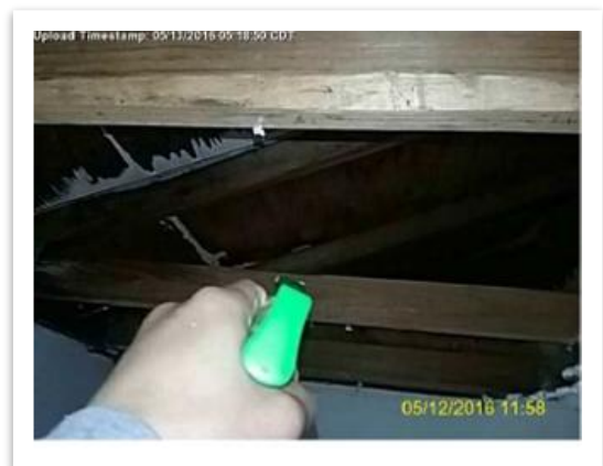
Treatment of studs with antimicrobial solution.
