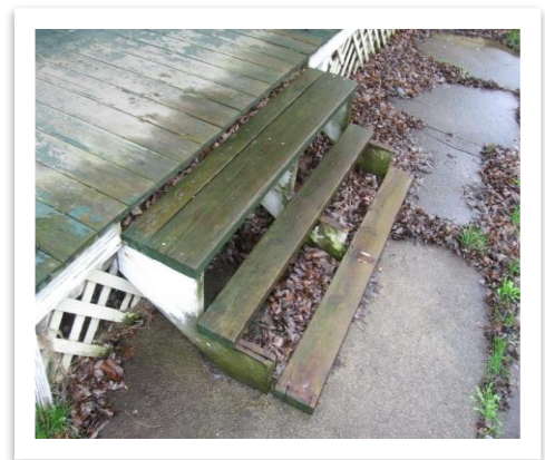
Damaged/missing treads and risers.
