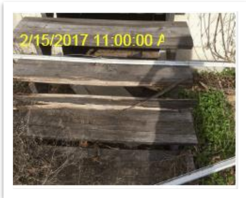
Damaged treads and risers.
