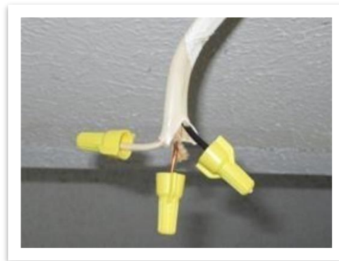
Example of Capping Wires
