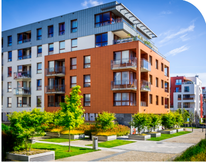
High-rise and mid-rise buildings with interior hallways
