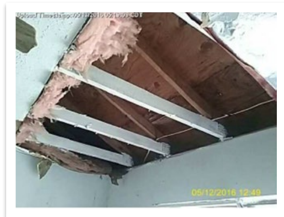
Treatment of studs with stain blocking primer.
