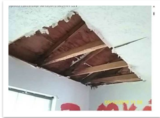
Removal of drywall and insulation.
