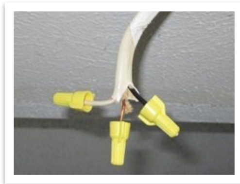
Example of Capping Wires
