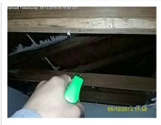
Treatment of studs with antimicrobial solution.
